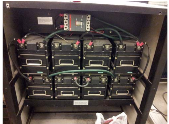
Fig. 1. Supercaps, mounted in rack
